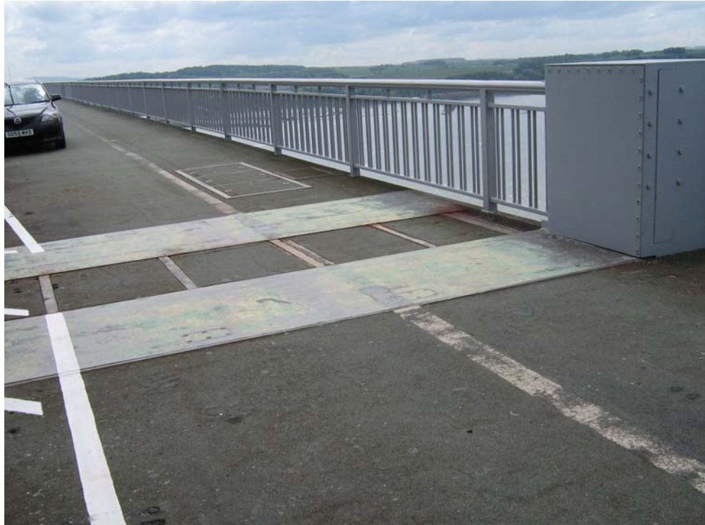
Photograph 3 – Sliding Plate Joint in Foot / Cycle Way
