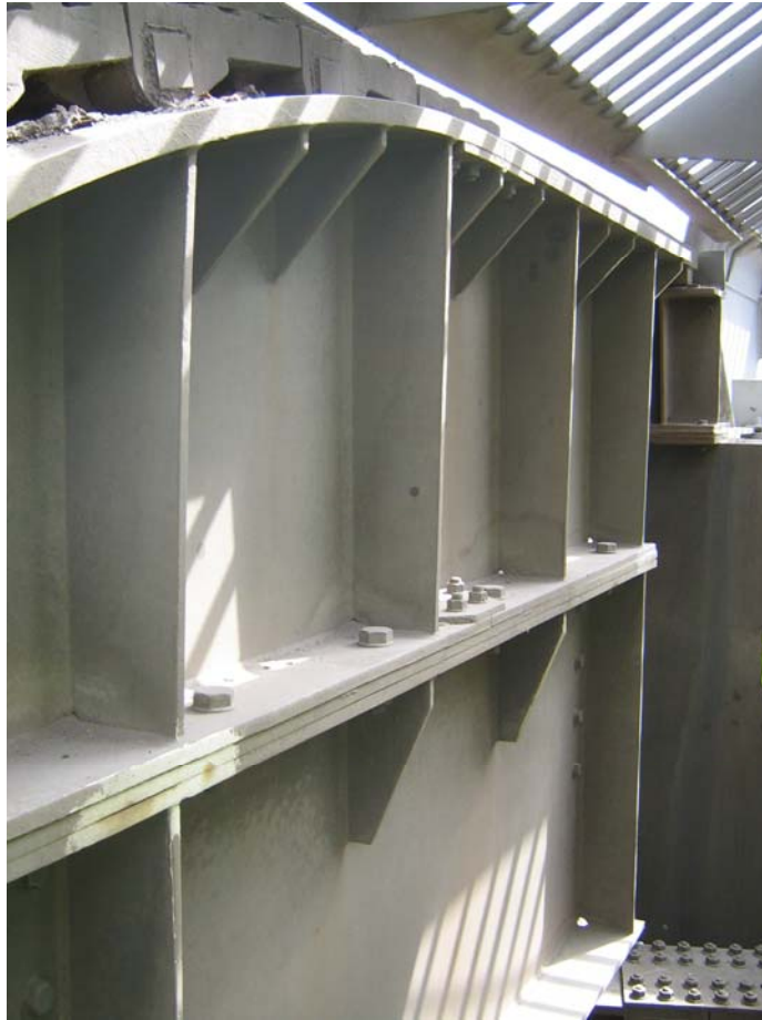
Photograph 1 – Roller Shutter Joint, View of Curved Link Plate Support Beam
