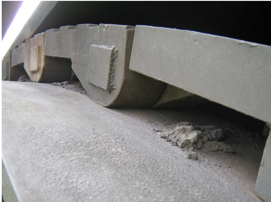
Photograph 2 – Roller Shutter Joint, Link Plate Train
