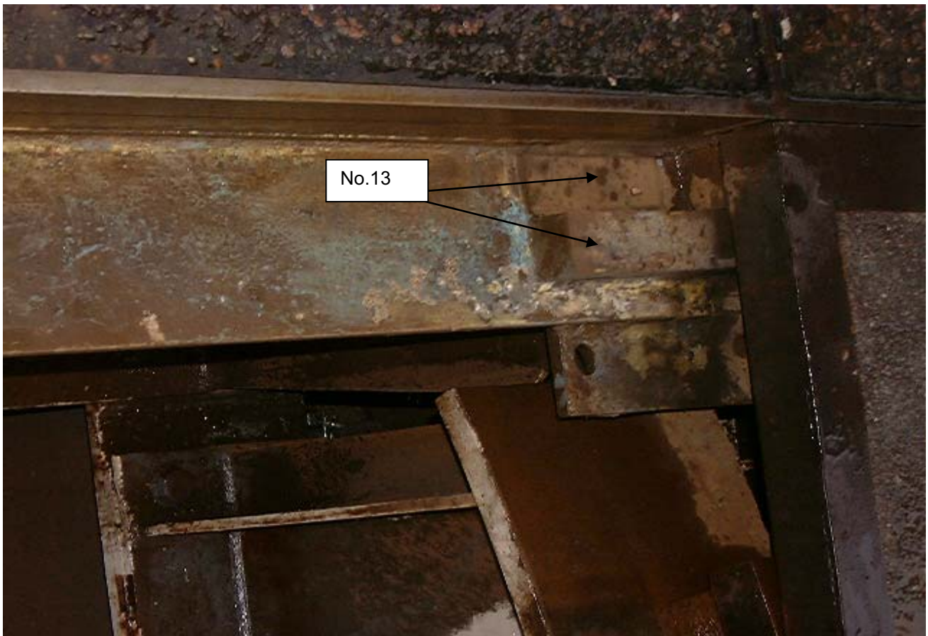
Photograph 5 – View of Tongue Plate Restraint Block
