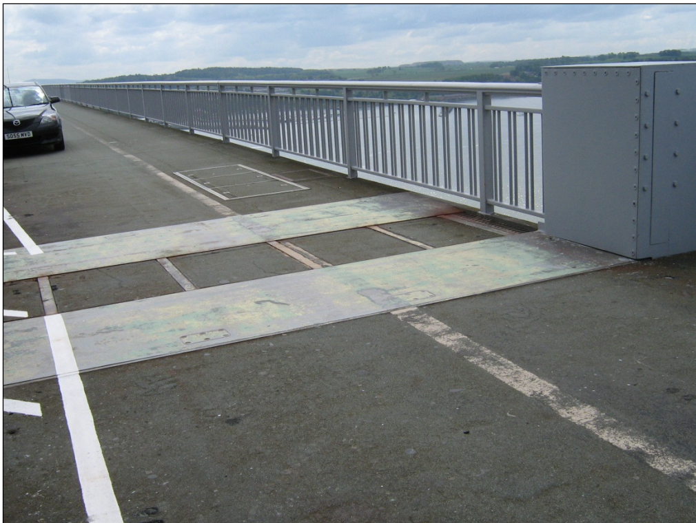
Figure 2 - Existing Foot / Cycleway Joint
