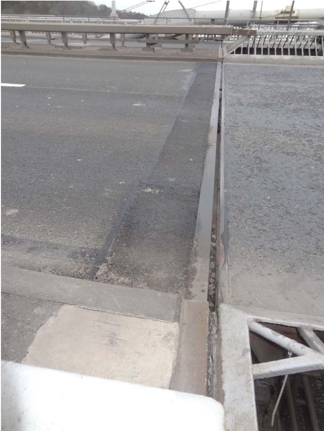
Figure B-1 View of Nosing Joint (North Side Tower, Northbound Carriageway)
