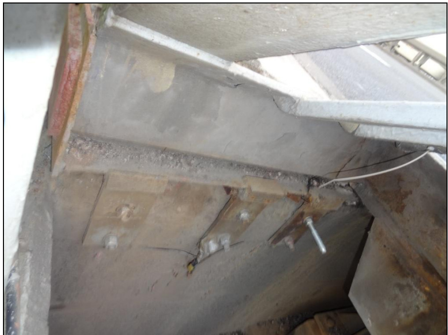
Figure 3-4 Additional Anchoring to the Steel Edging on the North Side Tower
