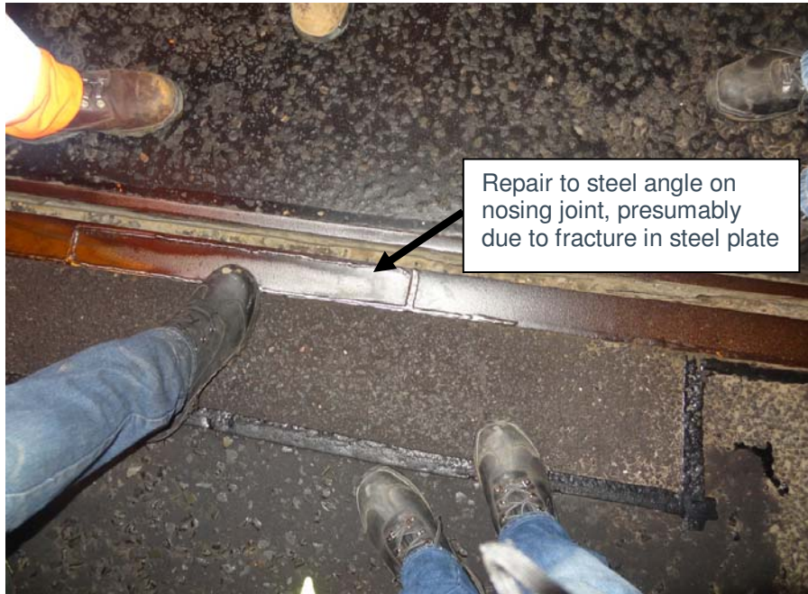
Figure 3-3 Local Repair to Steel Edging on North Side Tower
