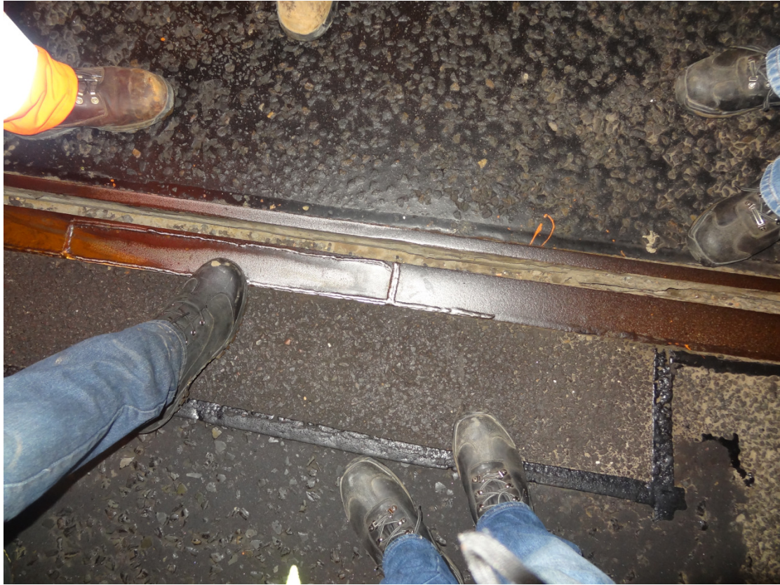
Figure B-4 View of Nosing Joint (Local Repair of Steel Edging Plate)
