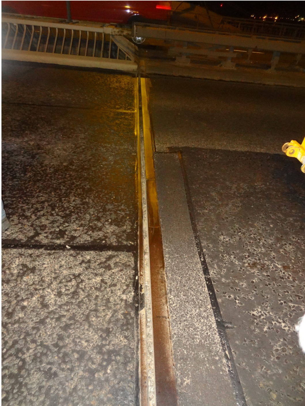
Figure B-2 View of Nosing Joint (South Side Tower, Southbound Carriageway)
