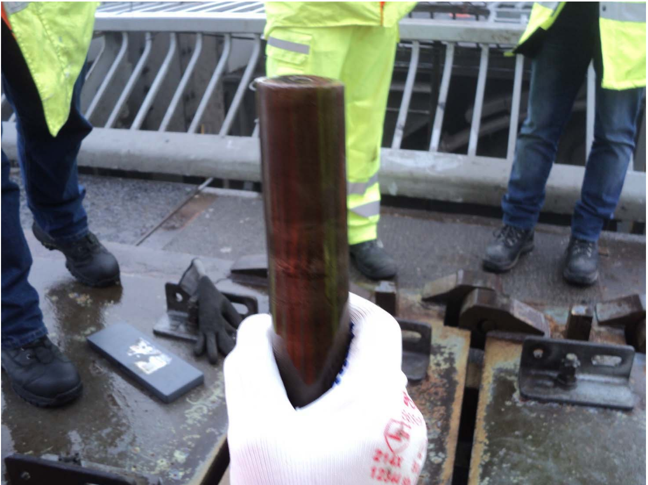
Photograph 15 – Hinge pins appear in good condition with little wear evident.
