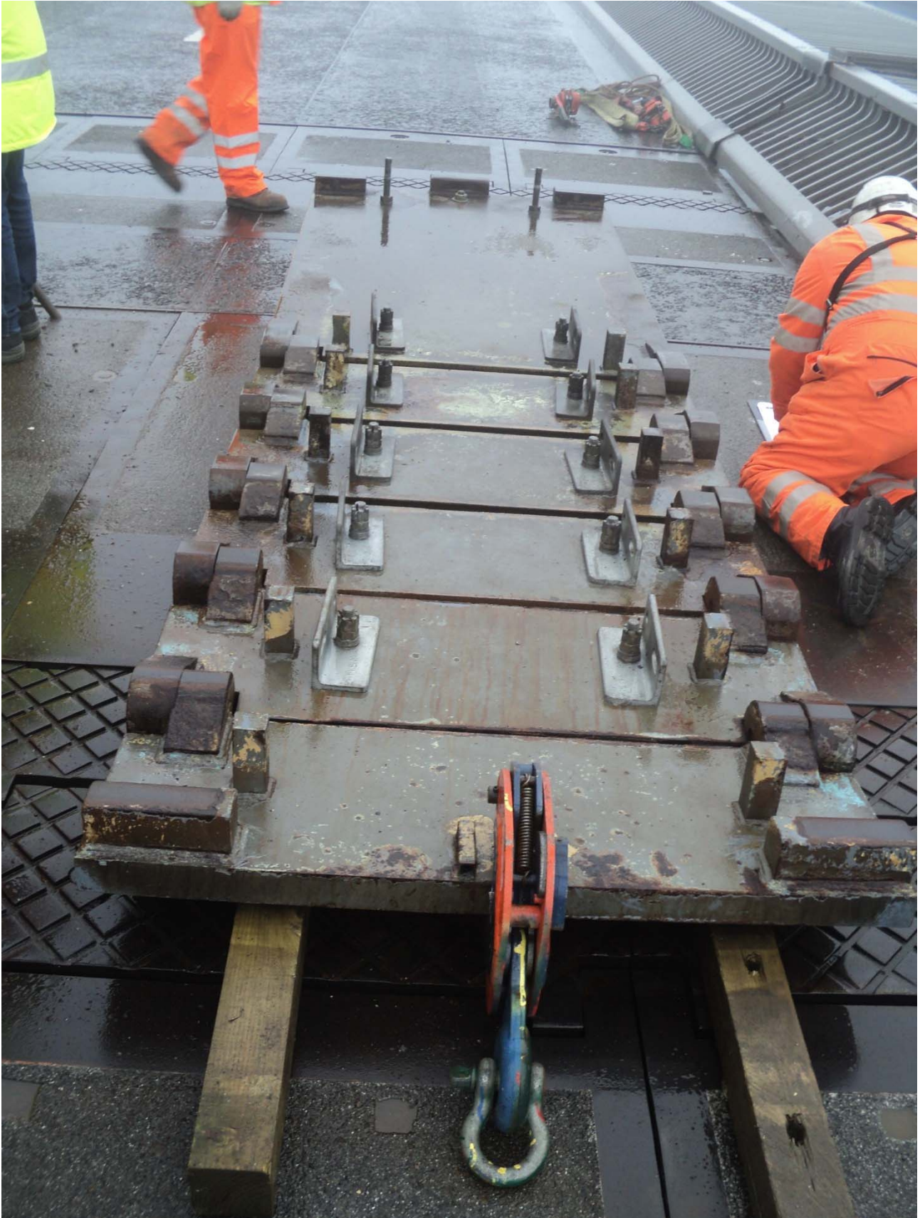
Photograph 1 – Overview of plate train, after removal and up-turned. Note failsafe linkages have been removed prior to lifting.
