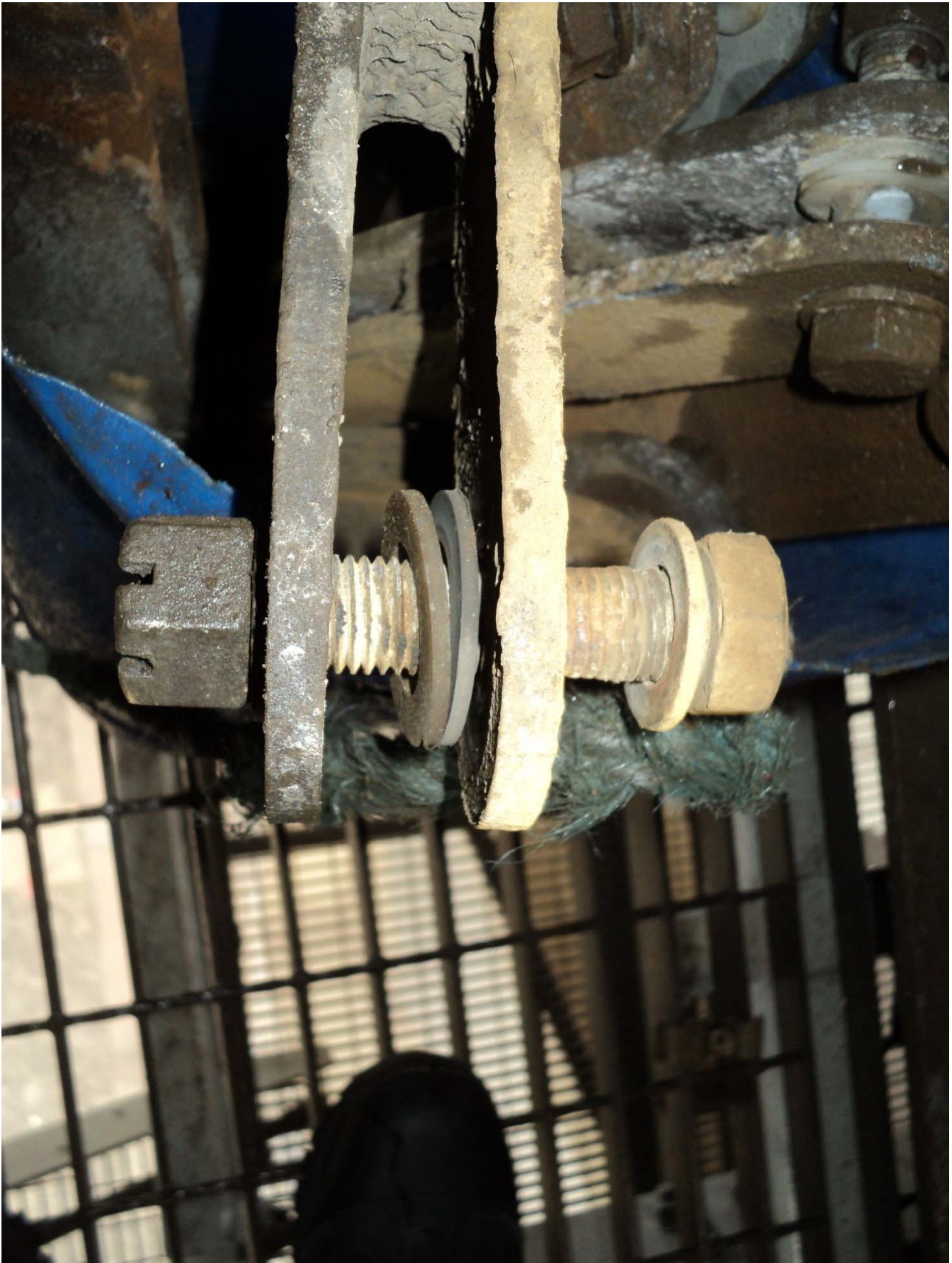
Photograph 17 – Wear on bolt thread of failsafe hinge linkage. Note bolt thread originally had nylon sleeve.
