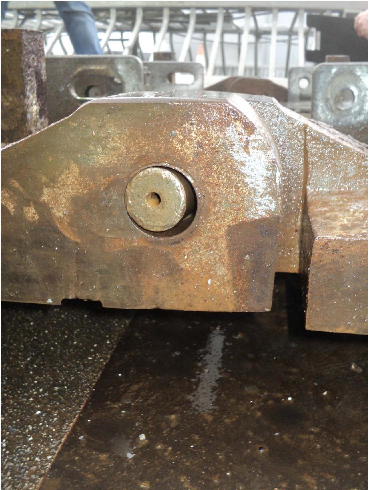
Photograph 3 – Typical wear to hinge and foot
