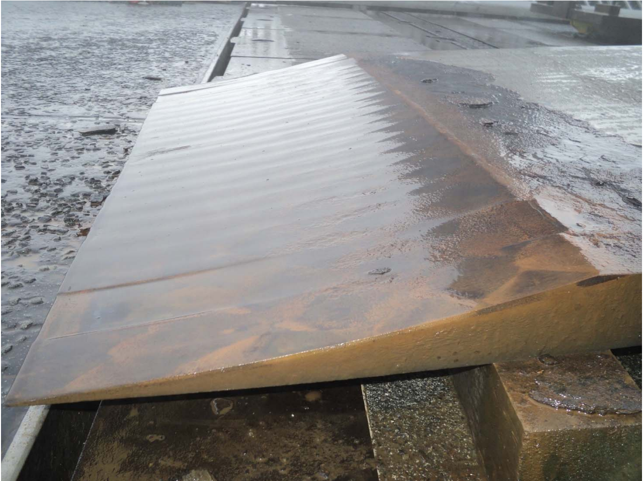
Photograph 6 – Worn tongue plate. Note thinning where grooves are worn where tongue plate rides over raised plate hinges. Tongue plates ends are trimmed to remove sharp edges created by wear.
