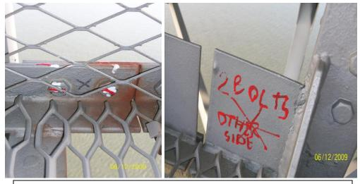
P.P.91 S.E. 2 SPLICE BOLTS LOOSE (EAST), 2 SPLICE BOLTS LOOSE (WEST).
