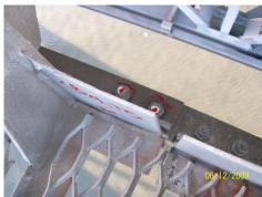
P.P.57 S.E. 2 SPLICE BOLTS LOOSE (EAST),2 SPLICE BOLTS LOOSE (WEST).
