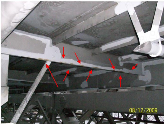
P.P. 65 N.W. LAST UPPER FRONT EXAMPLE OF TOUCHED UP AREAS SHOWING SIGNS OF BREAKDOWN
