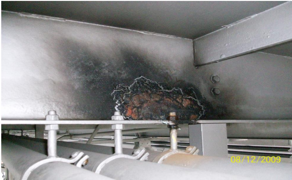
P.P.93 S.W. (1 ST BEAM NORTH OF P.P.) PAINT DAMAGE
