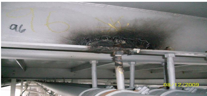
P.P.93 S.W. (1 ST BEAM NORTH OF P.P.) PAINT DAMAGE
