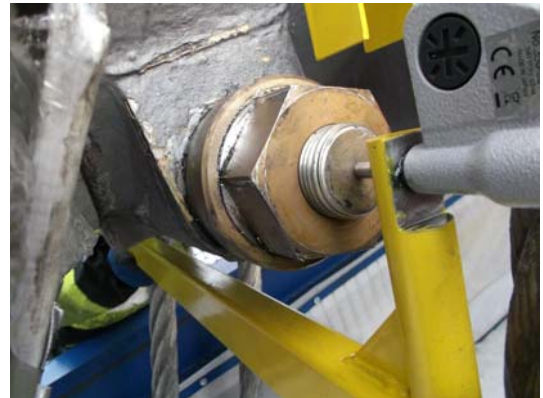
New bolt being measured
