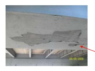
Localised area of paint breakdown on box girder soffit section, no 51 ( west )
