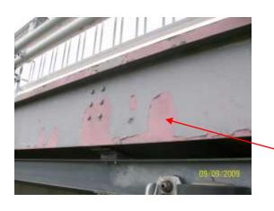
Areas of paint breakdown throughout viaduct on cycle track outer edge beam.
