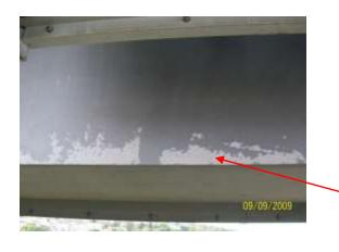
Areas of paint breakdown located box sections 32,33 & 34x. outer beams 130 x to 139x.
