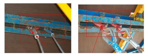
Beeche platform feeder cradle motor wires and safety wires are attached as shown above to a rectangular secured beam which is attached to the framework of the structure of the platform. Wires have fixed crimped captive hooks which are attached to GRADE. 8.8. M 24 mm bolts which are located and fixed through the lifting beams.
