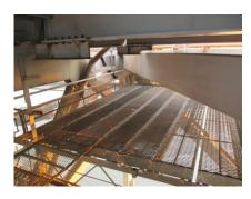
PP 50 - New half joint hard-ox packer system installed. Gaps appearing between packers & lower jaws of half joints. Slight deck panel movement evident. Fitted packers appear to be moving forward on jaws of half joint. Remains satisfactory A/T/O/I.
