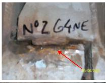
No.2 stringer 64 N.E., weld has been applied above and below, without welding the packer to the joint. This joint has not been successfully packed, as it is still banging.
