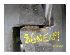
No.1 Stringer 86 N.E. joint has not been packed properly and still has movement.
