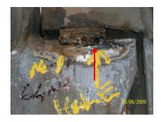
No.1 Stringer 64 N.E. Large hole at end of weld.
