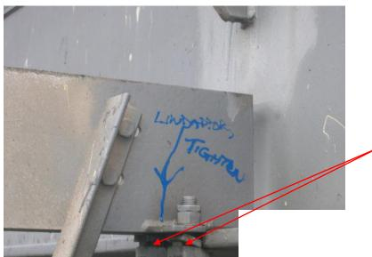
Walkway support bracket lindaptors on both e & w side of support beam require to be tightened movement no clamping .
