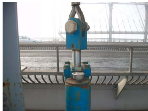
Dampener 15 south, main span side. 30 bar pressure ram extension 110mm
