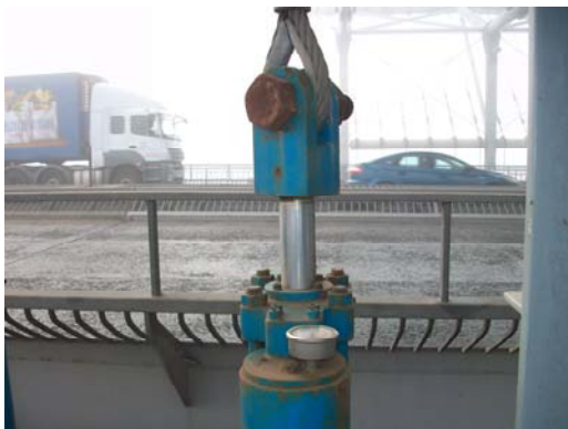
Dampener 16 south, main span side. 40 bar pressure, ram extension 142 mm.
