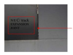
Grinding noise being generated by tower movement at time of inspection. Metal to metal.
