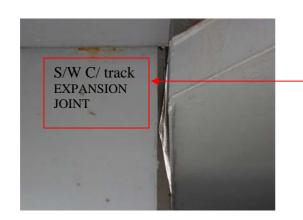
Gap differences between north east main tower and the south west main tower – main-span sides . Noise being generated by movement on the north east main tower side.
