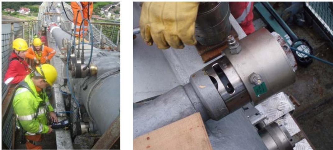
Fig 5.18: Hydraulic tensioning equipment as used to replace failed nuts
