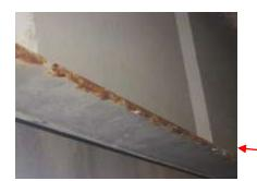
Areas of paint breakdown & corrosion evident on outrigger & crossbeam edges. & box girder face.
