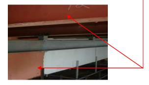
Areas of paint breakdown / unpainted box girder & outrigger beams.
