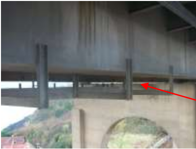
View of Redundant platforms located both East& West sides of boxes 44 & 44x.
