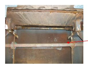
Bracer scaffold tube & fixings remain located between cell radius arms in every cell located on main-span & sidespan. require to be removed.
