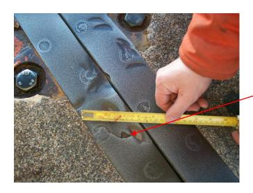
Surface plate located on main-span east. Damage and wear – down evident.
