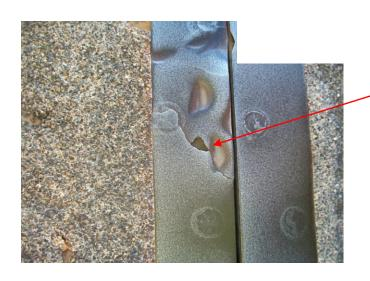
Surface plate located on main-span east. Damage and wear – down evident, Transverse weld crack approx 80- 100 mm .Requires to be repaired.
