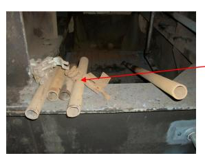
Tube & fitting off- cuts & fixings located on cell ledges, require to be removed.
