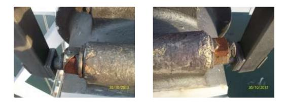
**Handstrand stanchions.** All hand-strands & bolt fixings throughout the main cable remain in a satisfactory condition. At PP 92 on the south east main span & north east main span the internal locking nuts on the east & west face in the underside of the hand-strand stanchion ( which is box section ) are not on the threaded bolt. ( could this been when handstrand stanchions were removed to allow main cable gantry access and not been put back in place ). Outer nuts remain in place and secure.
