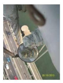
**<u>Cable bands sealant.</u>** : All the cable band sealant which is located on top & bottom half of the collars is in situ & remains in a satisfactory condition, however there are 7 locations where there are slight air leaks evident. South west side span. : - PP 18. ( north side ) South east side span. : - PP 34. 9 ( north side ) South east main span. : - PP 62, 66, 70 & 100 (all south side ) North east main span. : PP 68. ( north side )
