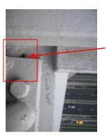
Photographs showing bolt holes & unpainted floor surface areas in North main tower top crossover internal
