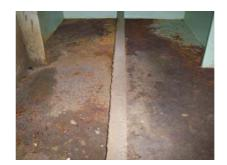
Photographs showing North main tower top crossover internal / external areas of water ingress. Bolts missing. Protective handrail fixing brackets.
