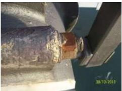
Handstrand Stanchions: All hand-strands & bolt fixings throughout the main cable remain in a satisfactory condition. At PP 92 on the south east main span & north east main span the internal locking nuts on the east & west face in the underside of the hand-strand stanchion (which is box section) are not on the threaded bolt. (this could have been when handstrand stanchions were removed to allow main cable gantry access and not been put back in place). Outer nuts remain in place and secure.
