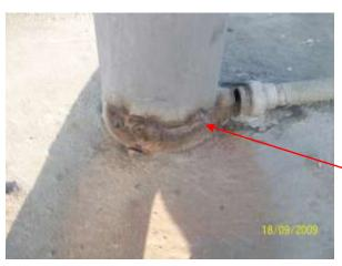
CORROSION EVIDENT AROUND PROTECTIVE MEMBRANE UPSTAND ON LIGHTING COLUMN BASE.
