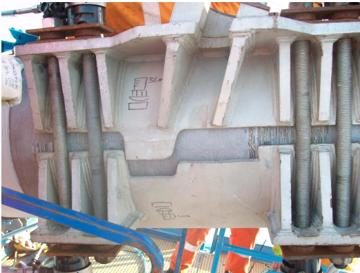
Photograph showing view of ( West side ) temporary cable band located on main cable.
