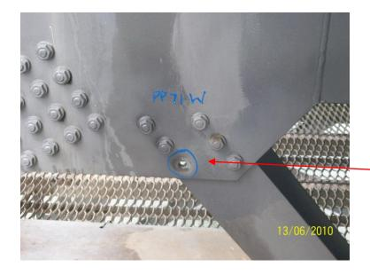
Missing bolt beam No 6 . on south face of cross girder PP71 (West. )
