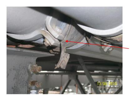
"A line "Tri-duct Expansion joint jubilee clips heavily corroded & broken, Require to be replaced on both E & W throughout Main-span PI. Area PP 68.5 to PP71.5.
