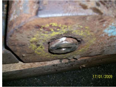
Position No. 8 External: Protruding pin, seized on inner lug. Pin ground down to ease reinstatement.
