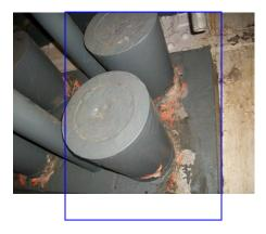
West side of crosshead block C6. Paint removed from west side and directly below top socket and on the west side of the bottom socket. ( No change from inspection date. (10.07.15.)
