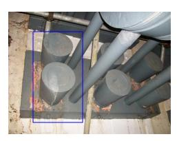
East side of crosshead block from area between poured sockets. Paint very brittle, cracking over whole Block evident. loss of adhesion. (No change from inspection date. (10.07.15.)
