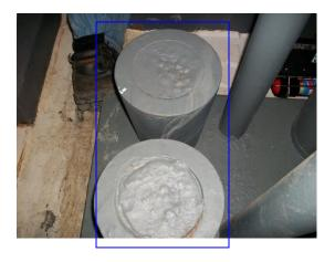
Sight area of zinc salts present on S/W corner of bottom socket. Area of paint breakdown evident. Top socket satisfactory. (No change from inspection date. . (10.07.15.)
