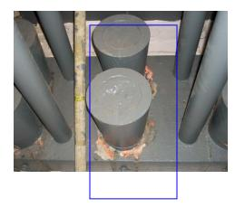
Centre of crosshead block C6. Paint removed from west side of socket and from directly below bottom socket. (No change from inspection date. (10.07.15.)
