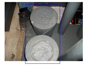
Sight area of zinc salts present on S/W corner of bottom socket. Area of paint breakdown evident. Top socket satisfactory. (No change from inspection date. (12.02.15.)
