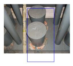
Centre of crosshead block C6. Paint removed from west side of socket and from directly below bottom socket. (No change from inspection date. (09.04.15.)
