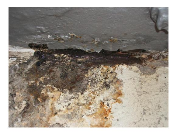
Small area of weeping over approx 200mm evident in centre where crosshead block meets anchorage face on <u>C6 . evidence of past</u> <u>staining but more prominent this weekly</u> <u>inspection. Localised.</u>
