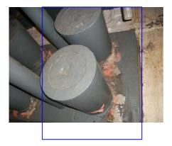
West side of crosshead block C6. Paint removed from west side and directly below top socket and on the west side of the bottom socket. ( No change from inspection date. (09.04.15.)
