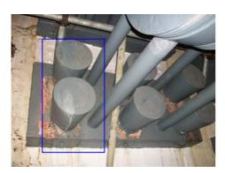
East side of crosshead block from area between poured sockets. Paint very brittle, cracking over whole Block evident. loss of adhesion. (No change from inspection date. (09.04.15.)
