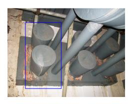
East side of crosshead block from area between poured sockets. Paint very brittle, cracking over whole Block evident. loss of adhesion. (No change from inspection date. (09.03.15.)
