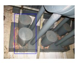
East side of crosshead block from area between poured sockets. Paint very brittle, cracking over whole Block evident. loss of adhesion. (No change from inspection date. (09.04.15.)
