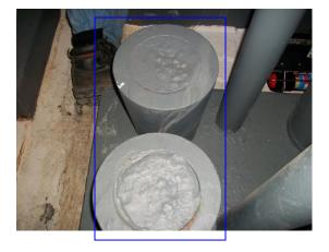
Sight area of zinc salts present on S/W corner of bottom socket. Area of paint breakdown evident. Top socket satisfactory. (No change from inspection date. (09.04.15.)
