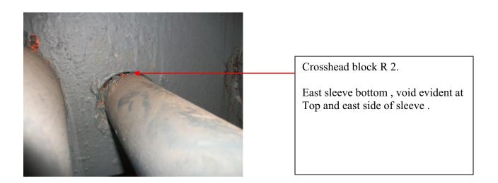
Voids evident on crosshead block R2. These were marked for indication of any movement or turning .
