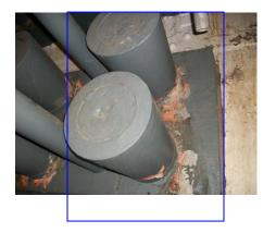
West side of crosshead block C6. Paint removed from west side and directly below top socket and on the west side of the bottom socket.
