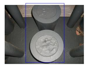
No paint missing from around top or bottom socket, no moisture evident.
