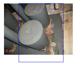
West side of crosshead block C6. Paint removed from west side and directly below top socket and on the west side of the bottom socket. ( No change from inspection date. (06.08.15.)
