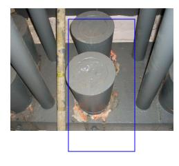
Centre of crosshead block C6. Paint removed from west side of socket and from directly below bottom socket. (No change from inspection date. (06.08.15.)
