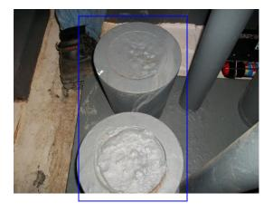
Sight area of zinc salts present on S/W corner of bottom socket. Area of paint breakdown evident. Top socket satisfactory. (No change from inspection date. . (06.08.15.)
