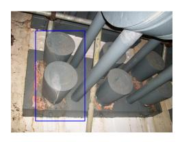
East side of crosshead block from area between poured sockets. Paint very brittle, cracking over whole Block evident. loss of adhesion. (No change from inspection date. (03.12.14.)
