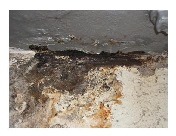
Small area of weeping over approx 200mm evident in centre where crosshead block meets anchorage face on C6. evidence of past staining but more prominent this weekly inspection. Localised.
