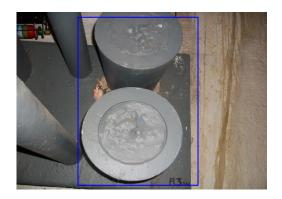
West side of crosshead block R3. paint removed from East & west side and directly below top socket.
