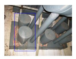
East side of crosshead block from area between poured sockets. Paint very brittle, cracking over whole Block evident. loss of adhesion. (No change from inspection date. (12.01.15.)
