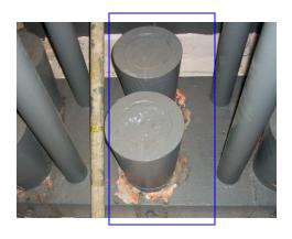
Centre of crosshead block C6. Paint removed from west side of socket and from directly below bottom socket. (No change from inspection date. (12.01.15.)
