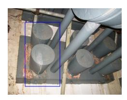
East side of crosshead block from area between poured sockets. Paint very brittle, cracking over whole Block evident. loss of adhesion. (No change from inspection date. (11.09.2015.)
