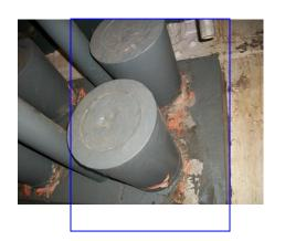
West side of crosshead block C6. Paint removed from west side and directly below top socket and on the west side of the bottom socket. (No change from inspection date. . (11.09.2015.)
