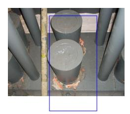
Centre of crosshead block C6. Paint removed from west side of socket and from directly below bottom socket. (No change from inspection date. . (11.09.2015.)
