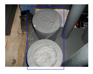
Sight area of zinc salts present on S/W corner of bottom socket. Area of paint breakdown evident.
