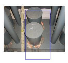
East side of crosshead block from area between poured sockets. Paint very brittle, cracking over whole Block evident. loss of adhesion. (No change from inspection date. (12.05.15.)
