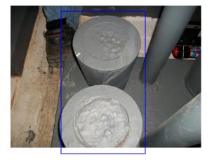
Sight area of zinc salts present on S/W corner of bottom socket. Area of paint breakdown evident. Top socket satisfactory. (No change from inspection date. . (12.05.15.)
