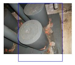
West side of crosshead block C6. Paint removed from west side and directly below top socket and on the west side of the bottom socket. ( No change from inspection date. (12.05.15.)
