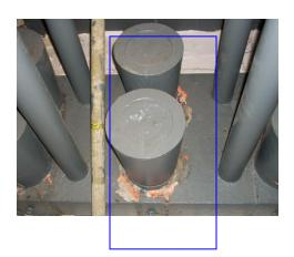
Centre of crosshead block C6. Paint removed from west side of socket and from directly below bottom socket. (No change from inspection date. (12.11.2015.)
