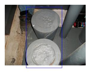
Sight area of zinc salts present on S/W corner of bottom socket. Area of paint breakdown evident.
