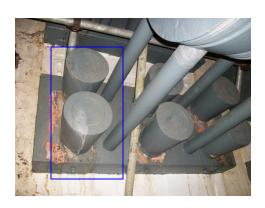
East side of crosshead block from area between poured sockets. Paint very brittle, cracking over whole Block evident. loss of adhesion. (No change from inspection date. (12.11.2015.)
