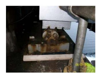
Photograph showing current status & condition of the North east viaduct box girder roller bearing & plinth from the east face.
