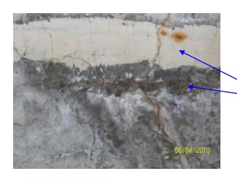
Discoloured area of concrete (possible sub-surface steel rebar beginning to show. Also transverse epoxy repair carried out pre- 1990.
