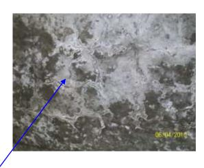
Views of heavy veinular cracking on deck soffit area.
