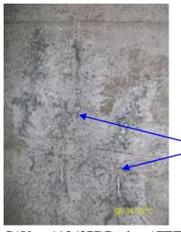
Two transverse cracks evident at affected area. Salts being discharged to deck soffit area.
