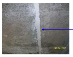
Transverse epoxy mortar repair carried out pre- 1990
