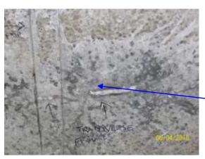
Another view of Transverse crack with Salts being discharged.
