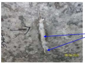
Salts being discharged from transverse cracks.
