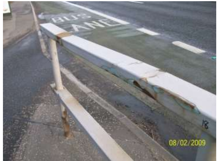
Top rail impact damage between positions 18 and 19.
