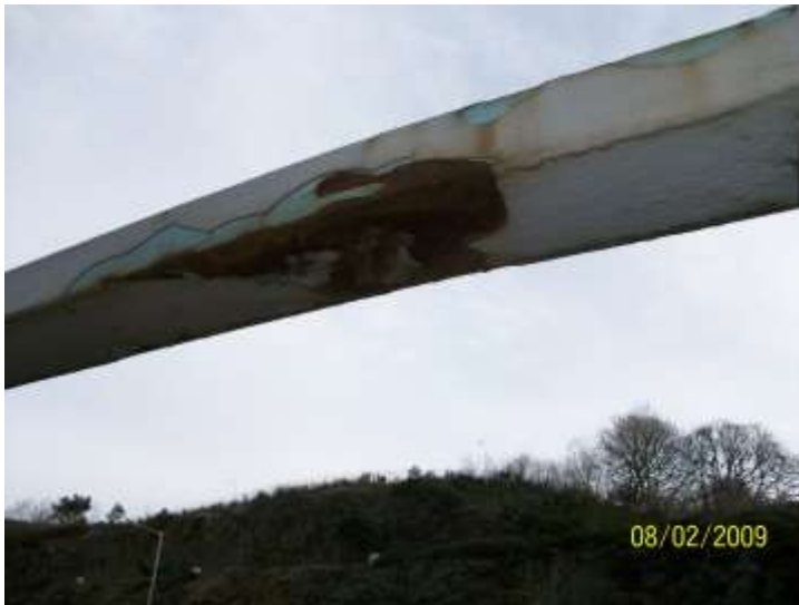
Top rail impact damage between positions 18 and 19.
