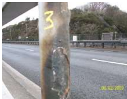
Example of corrosion.
