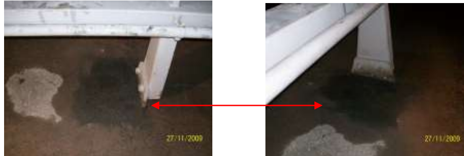
Photographs showing completion of surface repairs following completion of investigation / survey by consultants Flint & neill.
