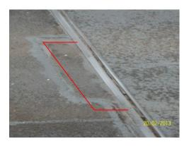
Photograph shows area where stiffener holding tang replacement was carried out. Noise/banging now evident. Probability is that further investigation / repair / replacement is required.
