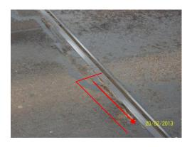
Excessive movement recorded on deck stiffener located on the North side of short deck panel Lane No 1. (Emergency temporary repair carried out by engineers 20. 02. 13).
