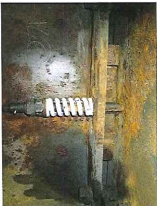
New spring fitted to rocker plate
