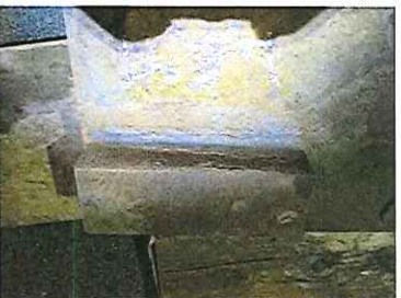
Rocker Plate End Bearing Blocks (East and West)
