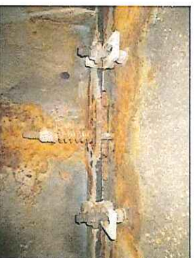
Condition of Rocker Plate and Springs
