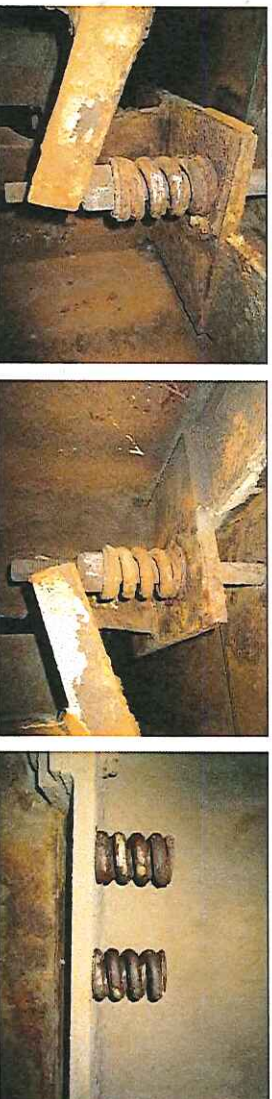
General condition of springs during pre-inspection
