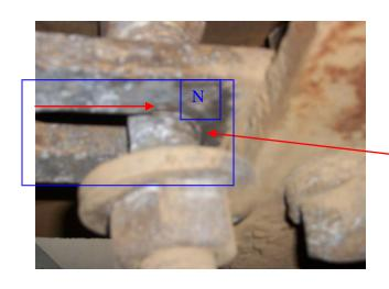
View from underside. This is probably down to vertical misalignment from topside on installation.
