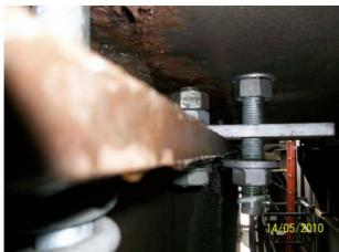
THE SIDE SPAN ROCKER LINK PLATE TO SUPPORT BEAM IS NOT FITTED TO DRAWING. LINK PLATES HAVE BEEN REEMED OUT TO ALLOW FOR ALIGNMENT WITH ROCKER PLATE HOLE. ALSO THE SPECIFIED 15mm CLEARANCE BETWEEN LINK PLATE AND WASHER IS NOW 25mm DUE TO CLASH WITH BEAM FLANGE.
