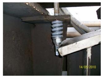
ON INSTALLATION OF THE SIDE SPAN TONGUE SPRING IT WAS DISCOVERED THAT THE FIXINGS CANNOT BE INSTALLED AS PER DRAWING, DUE TO A CLASH WITH THE RADIUS GIRDERS. THIS IS ILLUSTRATED IN THE PHOTOS. IF SECOND NUT IS TO BE INSTALLED TO DRAWING
