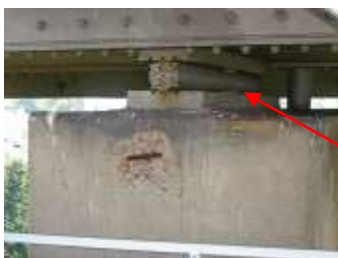
Roller bearing at S/E 6..
