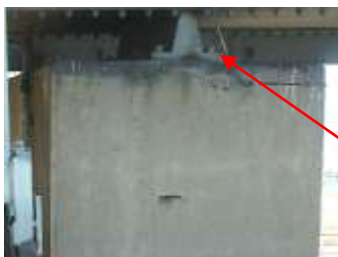
Pin bearing at S/E 2.
