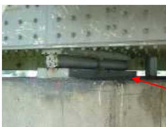
Roller bearing at S/E 4.
