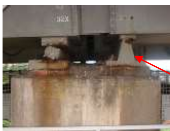
Roller & Pin bearing at S/E 3.
