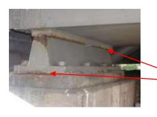
Paint breakdown & corrosion evident on Pin bearing.
