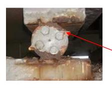
Example of. Roller bearing. Heavy corrosion & Paint breakdown.
